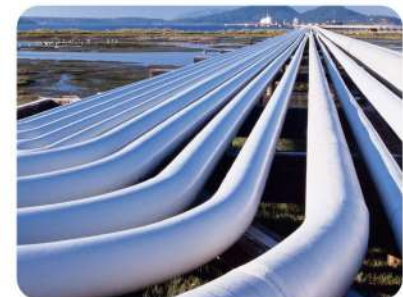
CROSS COUNTRY PIPELINE
